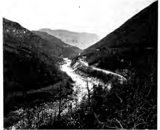
FIG. 4.—SUPPLY CANAL AT TUNNEL ENTRANCE.
